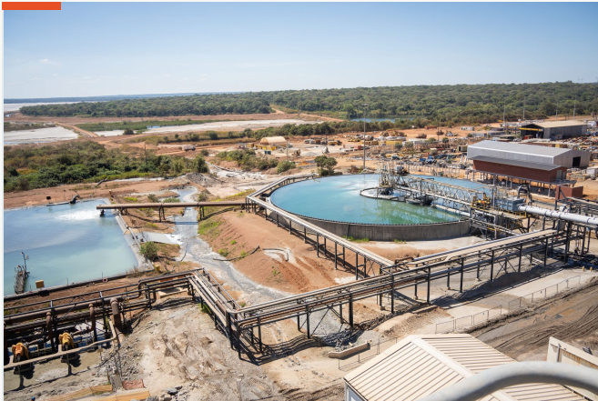
Plant overview and processing infrastructure.
